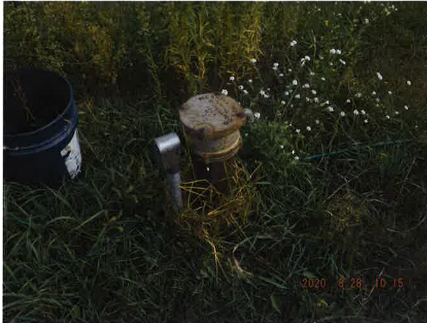
Figure B-2. Photograph of well pump and iron stained drop pipe
